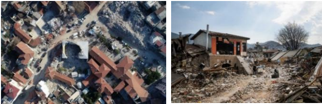
Figure 1. Areas destroyed in the Antakya earthquake
